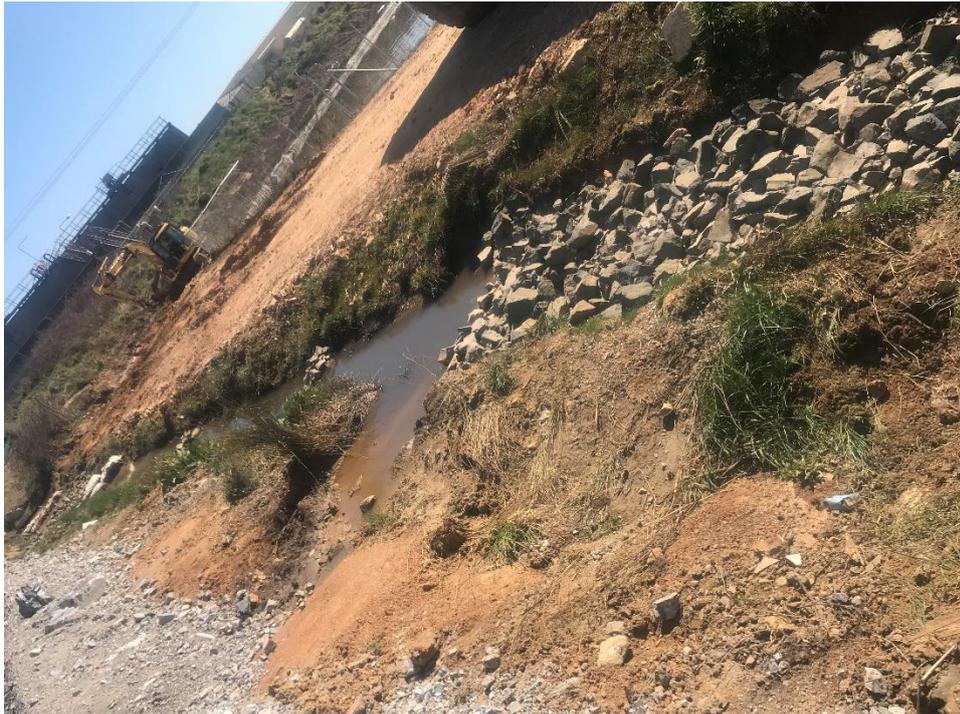
Image 1: Swale drain lined with scour rock
